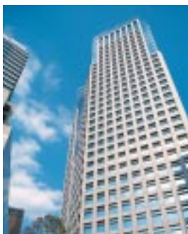
Garden Air Tower (Completed in February 2003/93,000m 2 )
