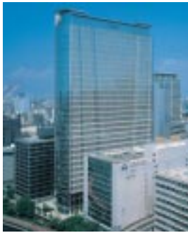
Nakanoshima Mitsui Building (Completed in August 2002/71,000m 2 )
