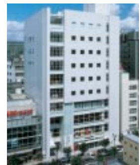
Ginza Namiki-dori Building (Completed in August 2002/9,000m 2 )
