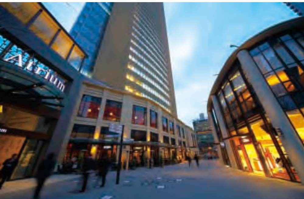
Akasaka Biz Tower (Office and retail facilities / Completed in March 2008)
