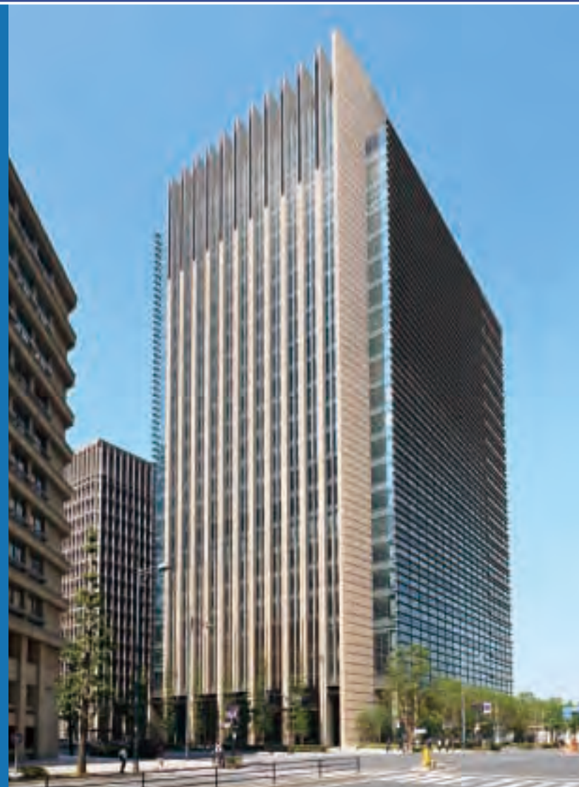
Sumitomo Mitsui Banking Corporation Head Office Building (Office building / Completed in July 2010)
