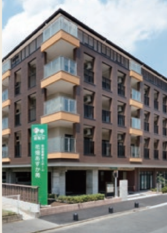
Hanahata Asuka-En (special nursing care home for senior citizens)* *This facility is the largest in Japan to be built using the 2x4 construction method (as of June 2018)
